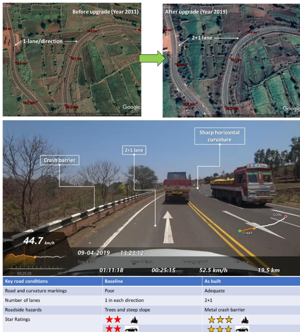
Figure 18: Improved road with 2+1 lane and curve delineation, Km 19.5 on the Belgaum–Yaragatti (SH-20) corridor in Karnataka
