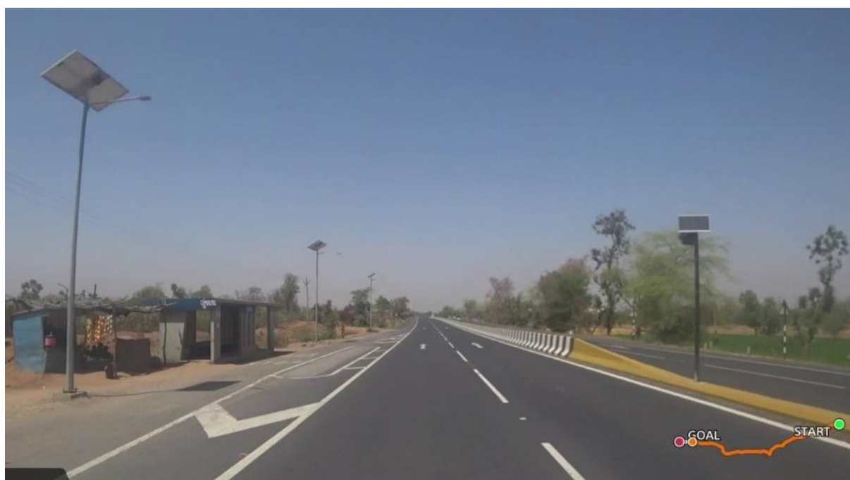
Figure 15: Example of Streetlight and delineation (road markings and signs) on the Mehsana–Himmatnagar (SH-55) corridor in Gujarat
