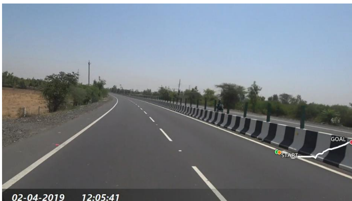
Figure 13: Concrete median barrier and paved shoulder on the Mehsana–Himmatnagar (SH-55) corridor in Gujarat
