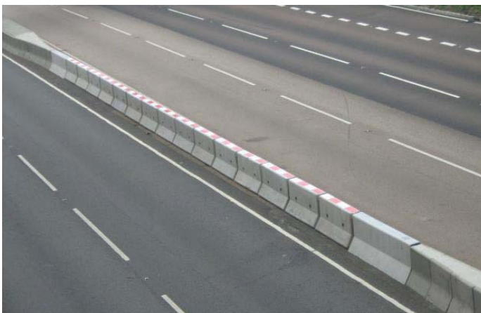
FIGURE 2.4.3.2 CONTINGENCY CROSSING WITH CRASHWORTHY SAFETY BARRIER
