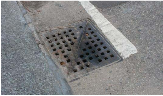
FIGURE 5.3.1.2 BICYCLE-FRIENDLY GULLY GRATING
