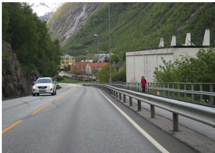
FIGURE 5.2.2.2 FOOTPATH PROTECTED BY SAFETY BARRIER ( driving is on the right side of the road )
