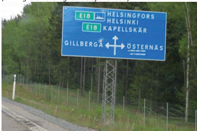
FIGURE 4.2.2.14 PASSIVELY SAFE SIGN STRUCTURE IN ALUMINIUM TRUSS
