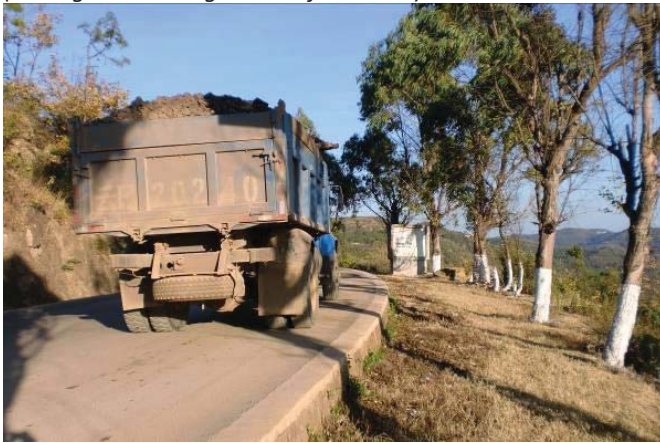
FIGURE 4.2.2.1 HAZARDOUS EDGE DROP DUE TO ROAD REHABILITATION (driving is on the right side of the road)
