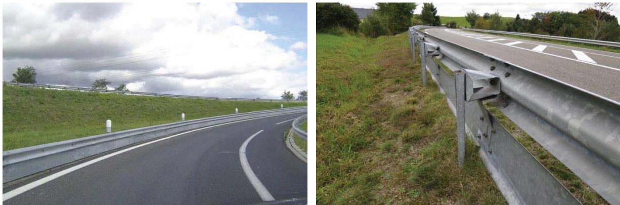
FIGURE 4.3.2.6 FLEXIBLE RUB-RAIL ON SAFETY BARRIER AT CURVES
