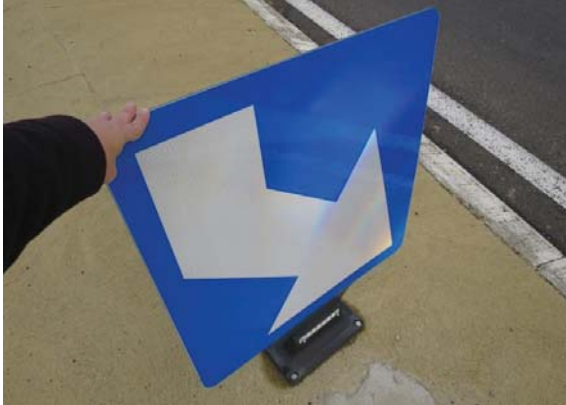
FIGURE 4.2.2.15 PASSIVELY SAFE SIGNS ON A TRAFFIC ISLAND
