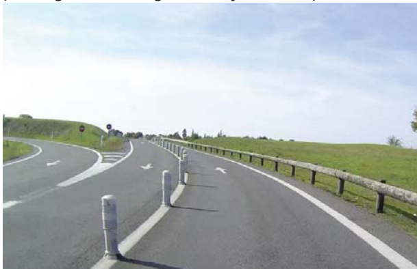
FIGURE 3.6.4.1 DELINEATORS AND REPEATED NO-ENTRY SIGN AT A GRADE-SEPARATED INTERSECTION (driving is on the right side of the road)
