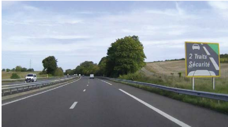
FIGURE 6.3.1.2 GAPS ON SHOULDER EDGE LINES SERVING AS MARKERS
