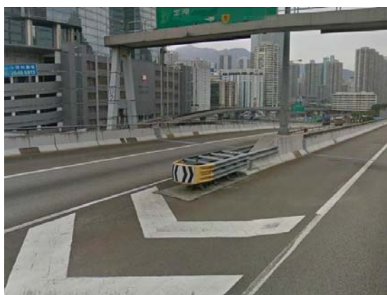
FIGURE 4.3.6.1 REDIRECTIVE CRASH CUSHION FOR NARROW (LEFT) AND WIDE (RIGHT) DIVERGE GORES (source: Traffic Safety System (HK) Limited) (driving is on the left side of the road)
