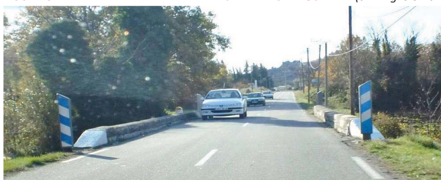
FIGURE 6.2.2.4 HAZARD MARKERS AHEAD OF A CULVERT (driving is on the right side of the road)
