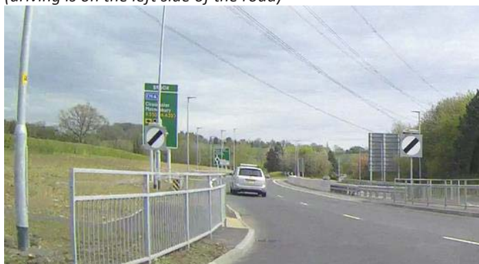
FIGURE 5.2.5.3 POTENTIAL MASKING OF WAITING AREA AT A CROSSING (driving is on the left side of the road)
