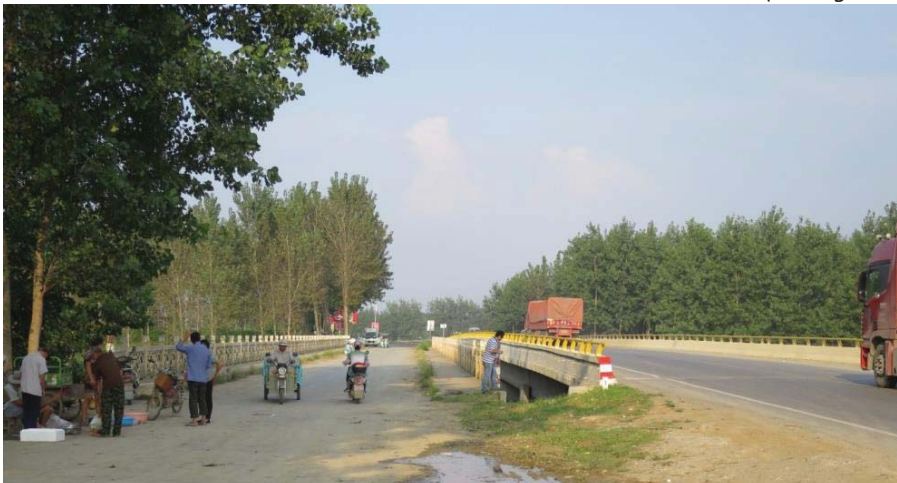
FIGURE 5.3.2.7 REUSE OF AN OLD BRIDGE FOR SLOW VEHICLES (driving is on the right side of the road)
