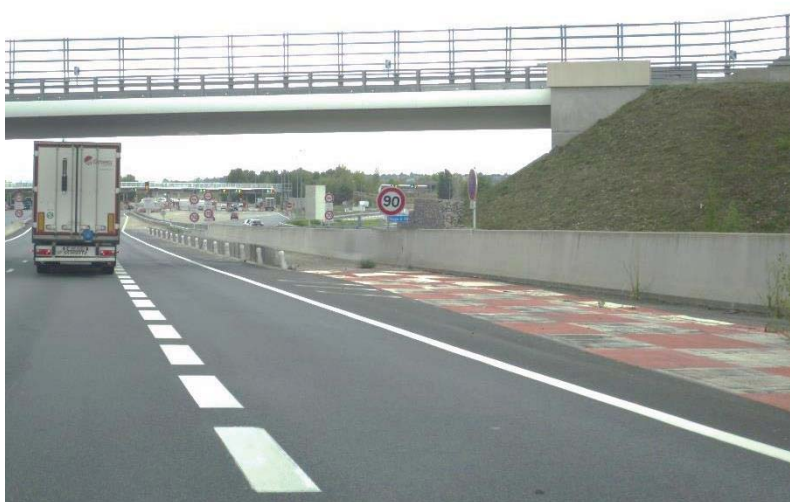
FIGURE 2.2.8.4 PARALLEL ESCAPE RAMP (driving is on the right side of the road)
