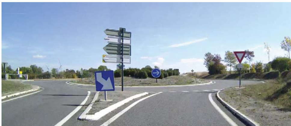
FIGURE 3.3.1.8 MASKING OF ROUTE CONTINUITY ON THE ROADSIDE OF A ROUNDABOUT
