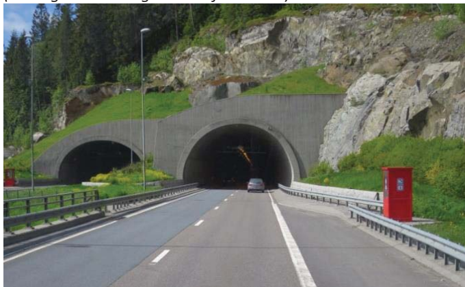
FIGURE 8.2.4.3 DOUBLE SAFETY BARRIERS AND ACCESS OPENING AT TUNNEL ENTRANCE
