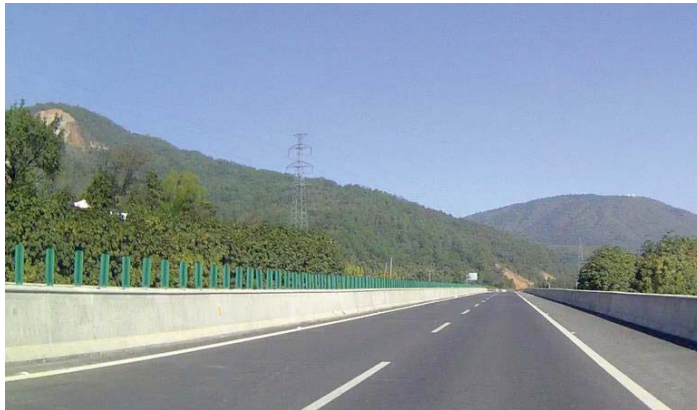
FIGURE 6.2.3.2 SAFETY BARRIER MOUNTED ANTI-GLARE SCREENS (driving is on the right side of the road)
