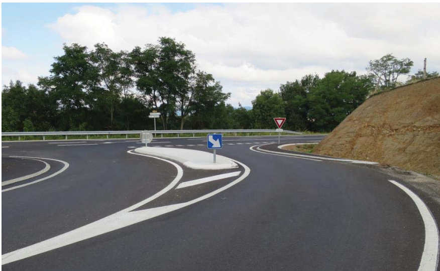
FIGURE 3.2.3.2 SIDE ROAD CHANNELIZING ISLANDS AT A CROSSROAD INTERSECTION (driving is on the right side of the road)
