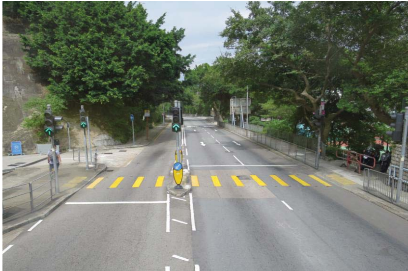
FIGURE 5.2.3.3 STANDALONE SIGNALISED CROSSING
