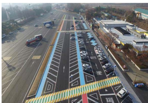
FIGURE 2.3.4.2 SEGREGATION OF HEAVY AND LIGHT VEHICLES, PEDESTRIAN PATHS AND TRAFFIC CALMING AT AN EXPRESSWAY SERVICE AREA IN THE REPUBLIC OF KOREA (driving is on the right side of the road)
