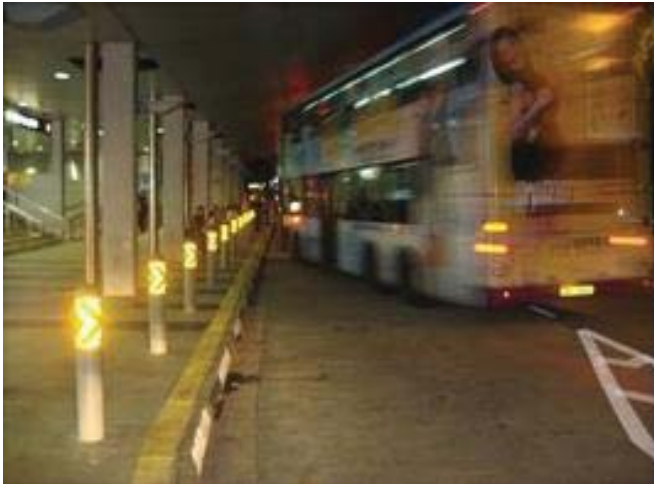
FIGURE 2.3.5.3 PASSIVELY SAFE BOLLARDS AT A BUS STOP IN SINGAPORE
