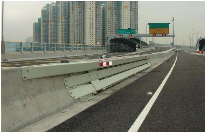
FIGURE 2.4.3.1 EMERGENCY CROSSING WITH CRASHWORTHY BARRIER GATE
