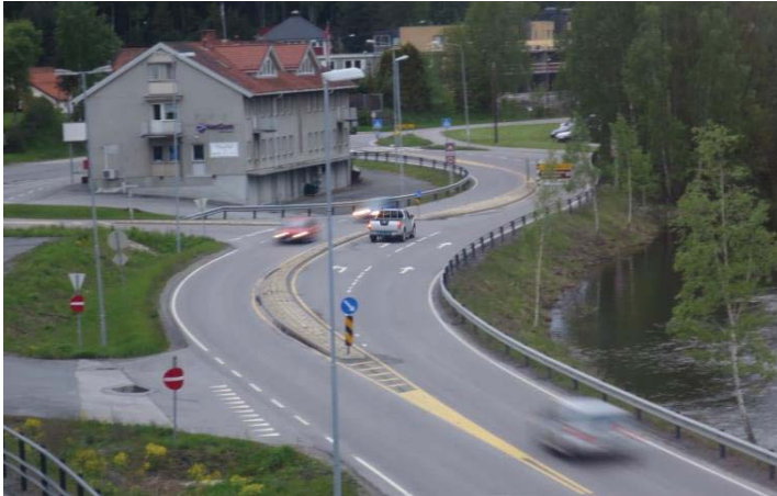
FIGURE 3.2.5.1 TYPICAL PROTECTED OFFSIDE TURN LANE WITH PHYSICAL TRAFFIC ISLANDS (driving is on the right side of the road)
