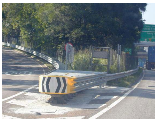
FIGURE 4.3.6.1 REDIRECTIVE CRASH CUSHION FOR NARROW (LEFT) AND WIDE (RIGHT) DIVERGE GORES (source: Traffic Safety System (HK) Limited) (driving is on the left side of the road)
