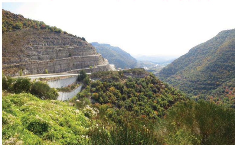
FIGURE 2.2.2.3 A PRIMARY ROAD ON DIFFICULT SECTIONS WITH EXTENSIVE EARTHWORKS
