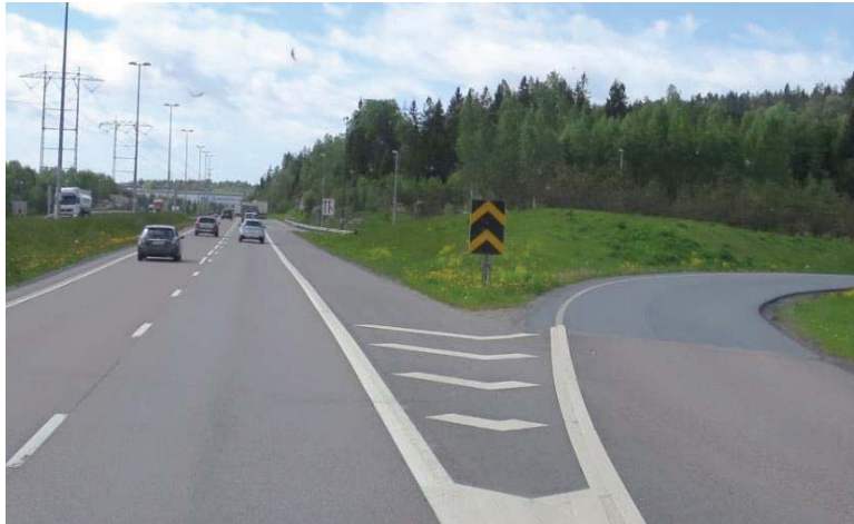
FIGURE 4.2.4.1 DIVERGE GORE IN CLEAR ZONE WITH MARKER SIGN ON PASSIVELY SAFE POST (driving is on the right side of the road)
