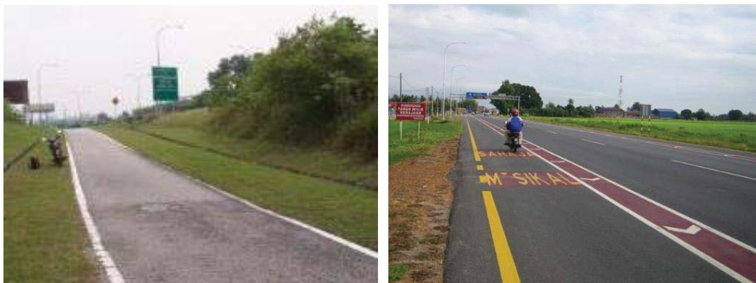
FIGURE 5.3.4.1 EXCLUSIVE MOTORCYCLE LANE (LEFT) AND NON-EXCLUSIVE MOTORCYCLE LANE (RIGHT) (Ref: iRAP) ( driving is on the left side of the road )
