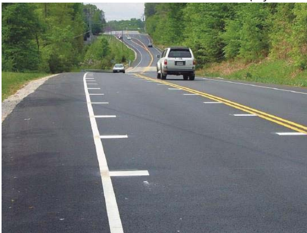
FIGURE 5.4.2.6 OPTICAL SPEED BARS (ref: FHWA, US, driving is on the right side of the road)
