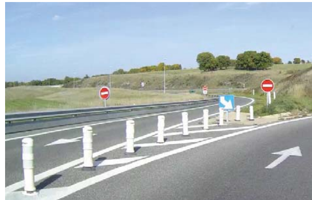
FIGURE 3.6.4.1 DELINEATORS AND REPEATED NO-ENTRY SIGN AT A GRADE-SEPARATED INTERSECTION (driving is on the right side of the road)
