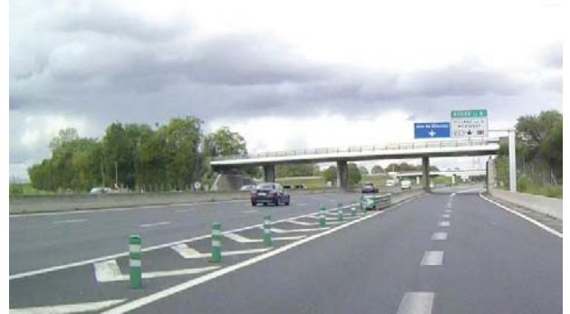
FIGURE 6.2.2.6 DELINEATORS AT DIVERGE GORES (driving is on the right side of the road)
