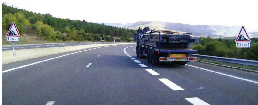
FIGURE 2.2.8.5 DOWNHILL AUXILIARY LANE ON A PRIMARY ROAD (driving is on the right side of the road)
