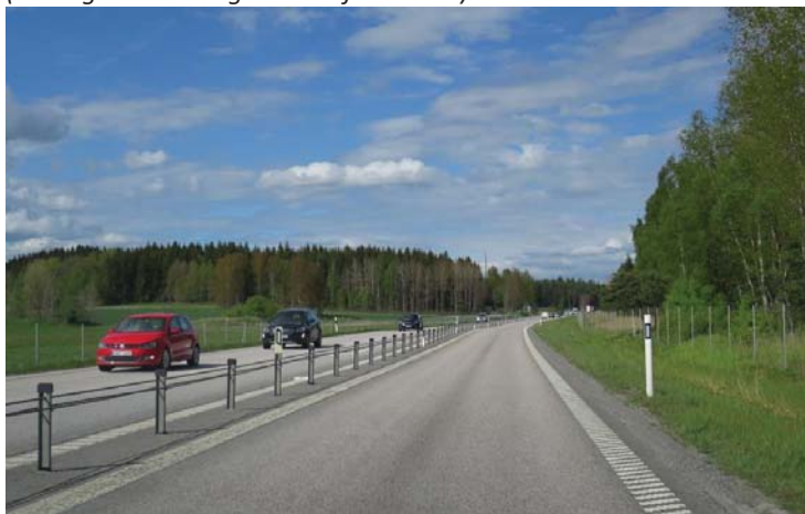
FIGURE 2.2.5.3 “2+1” ROAD WITH MEDIAN SAFETY BARRIER
