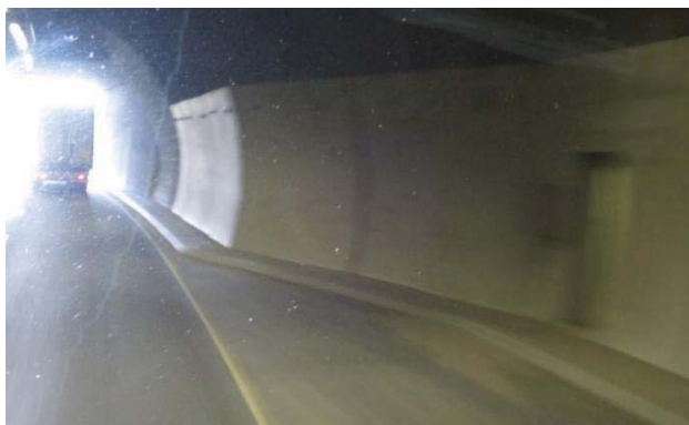
FIGURE 8.2.4.1 TERMINATION OF EMERGENCY LAYBY INSIDE TUNNEL
