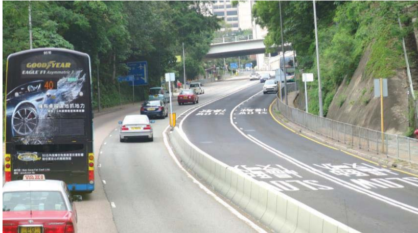
FIGURE 2.5.1.2 HIGH FRICTION SURFACING ON A DOWNHILL GRADE (driving is on the right side of the road)
