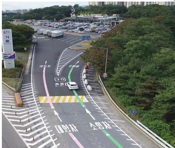
FIGURE 2.3.4.1 GUIDANCE AND TRAFFIC CALMING AT THE ENTRANCE TO AN EXPRESSWAY SERVICE AREA IN THE REPUBLIC OF KOREA (driving is on the right side of the road)
