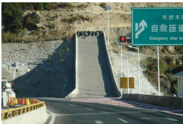
FIGURE 2.2.8.2 SLIP ROAD ESCAPE RAMP WITH A STEEP UPHILL ARRESTER BED
